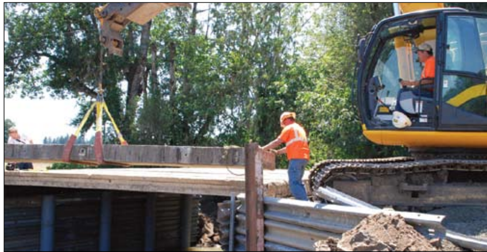
Benton County road workers construct a bridge on Stow Pit Road.
