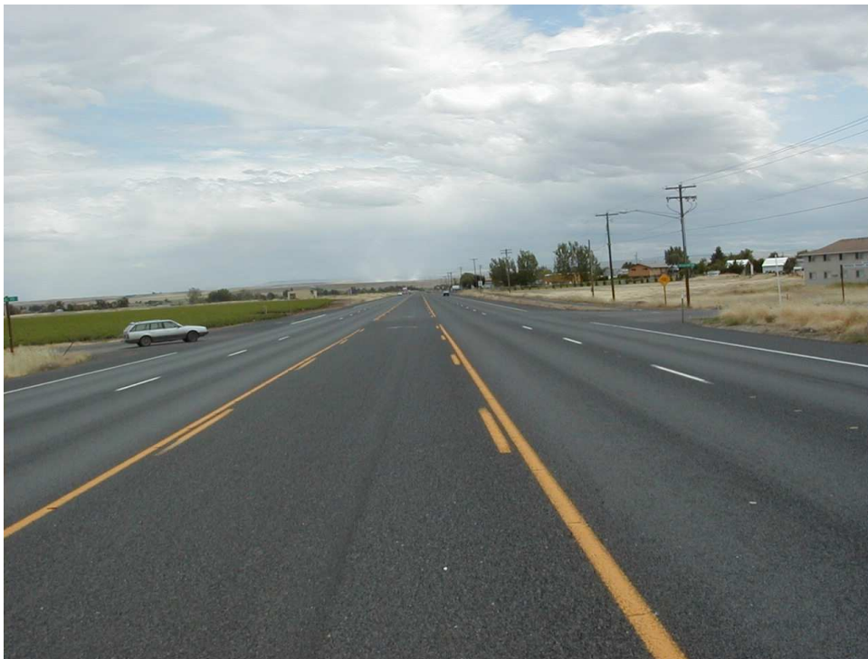
2. Looking south from 150 feet north of Rosalynn Drive.
